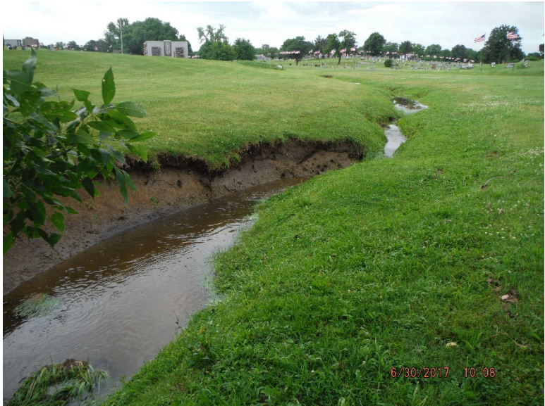
Photo 3.4.1 Outfall #6 Facing South/Southeast
