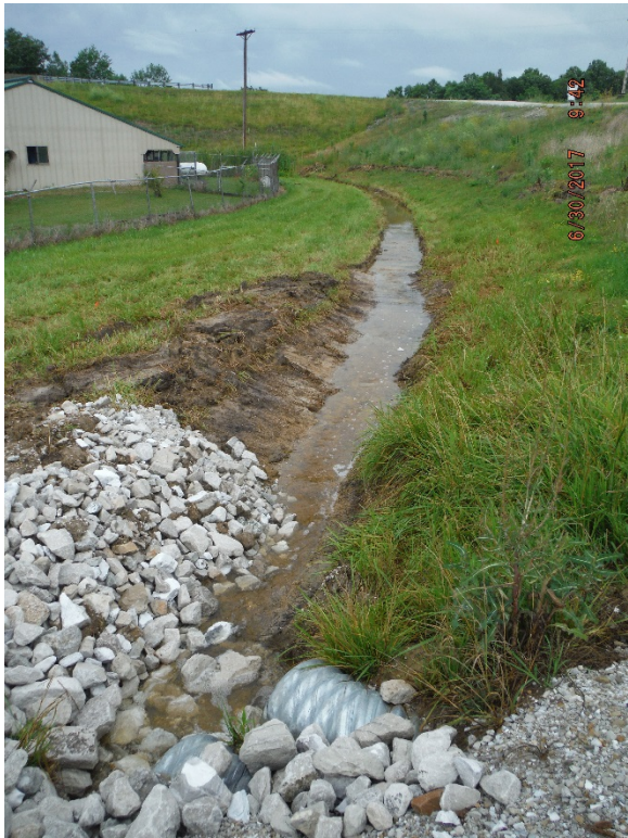
Photo 3.4.2 Outfall #7 Facing East
