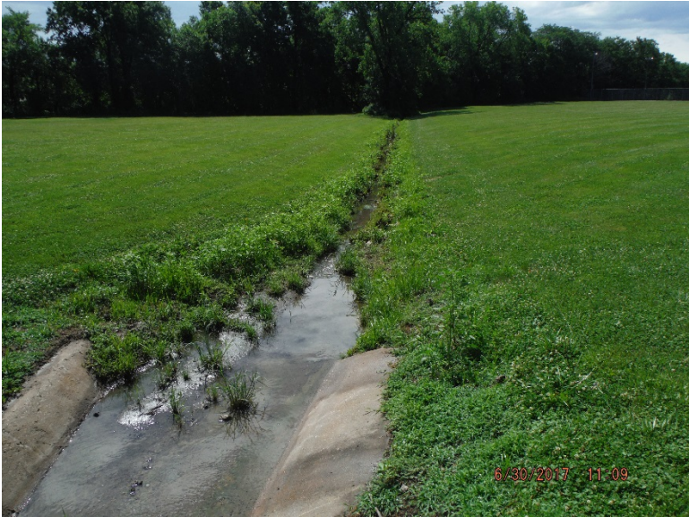
Photo 3.5.2 Outfall #8 Facing Southeast
