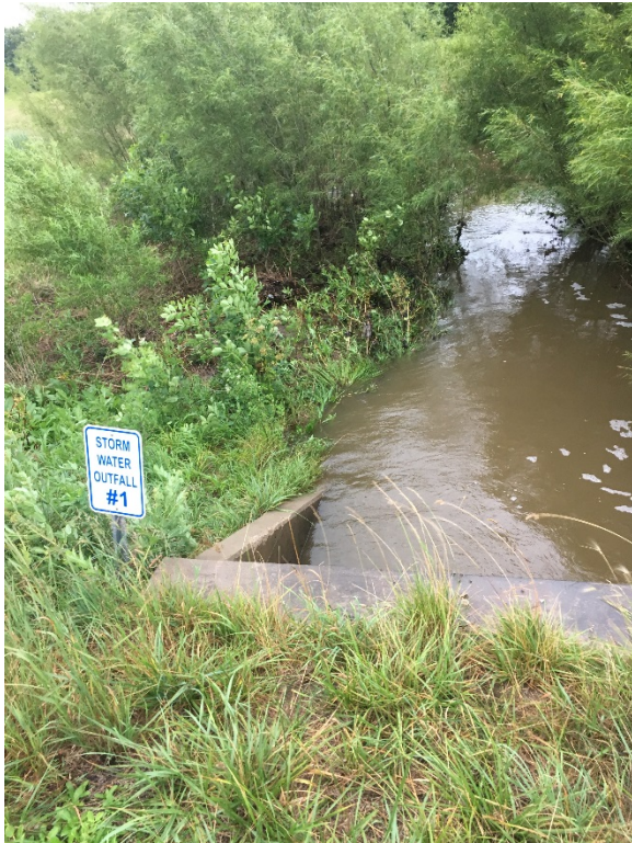
Photo 3.1.1 Existing Outfall #1 Facing Northeast
