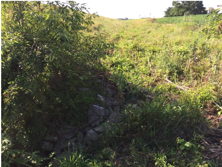
Photo 3.3.3 Outfall #4 Facing South
