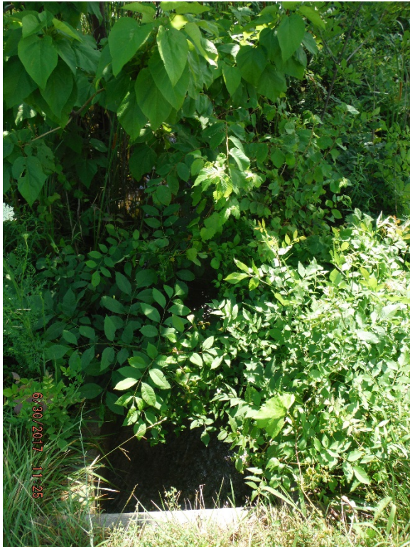
Photo 3.5.4 Outfall #10 Facing East (downstream)
