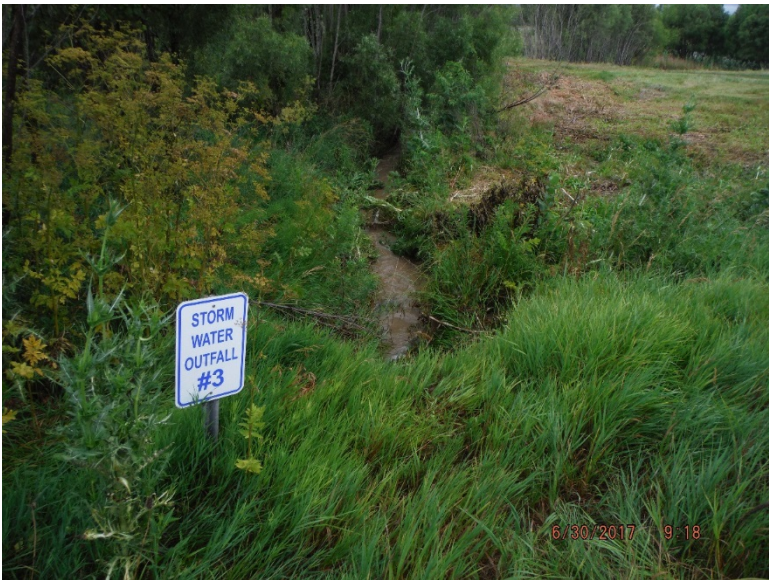
Photo 3.3.1 Existing Outfall #3 Facing Southeast
