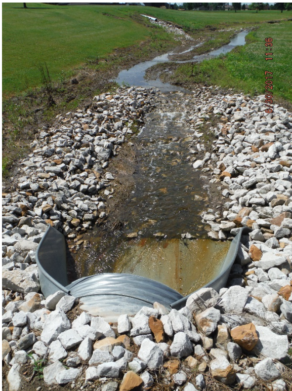
Photo 3.5.5 Outfall #11 Facing South
