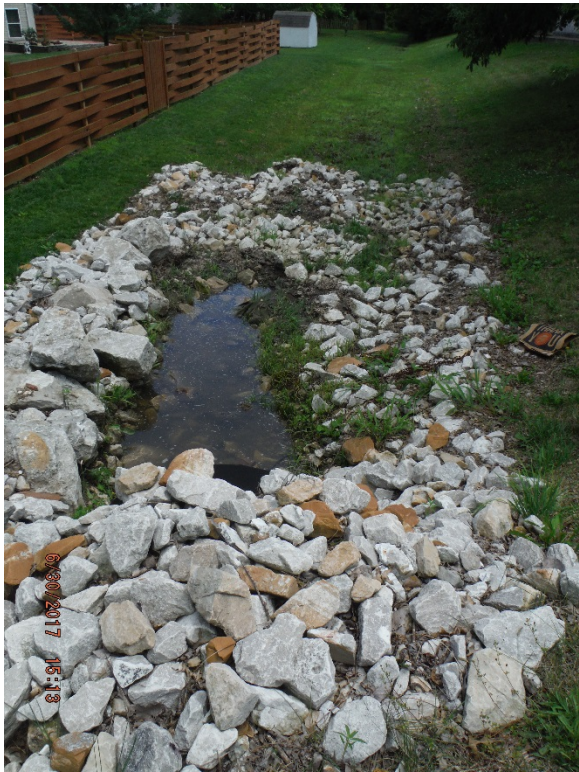
Photo 3.6.3 Outfall #14 Facing South/Southeast
