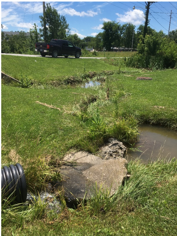
Photo 3.8.2 Outfall #19 Facing Southwest
