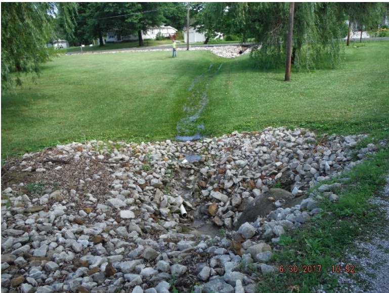
Photo 3.5.3 Outfall #9 Facing Northwest
